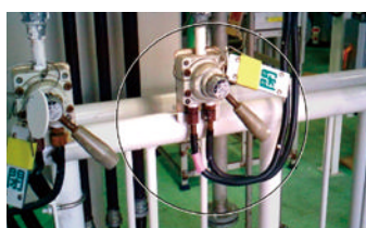
Air leaking from a connector (right: leakage detection image)
